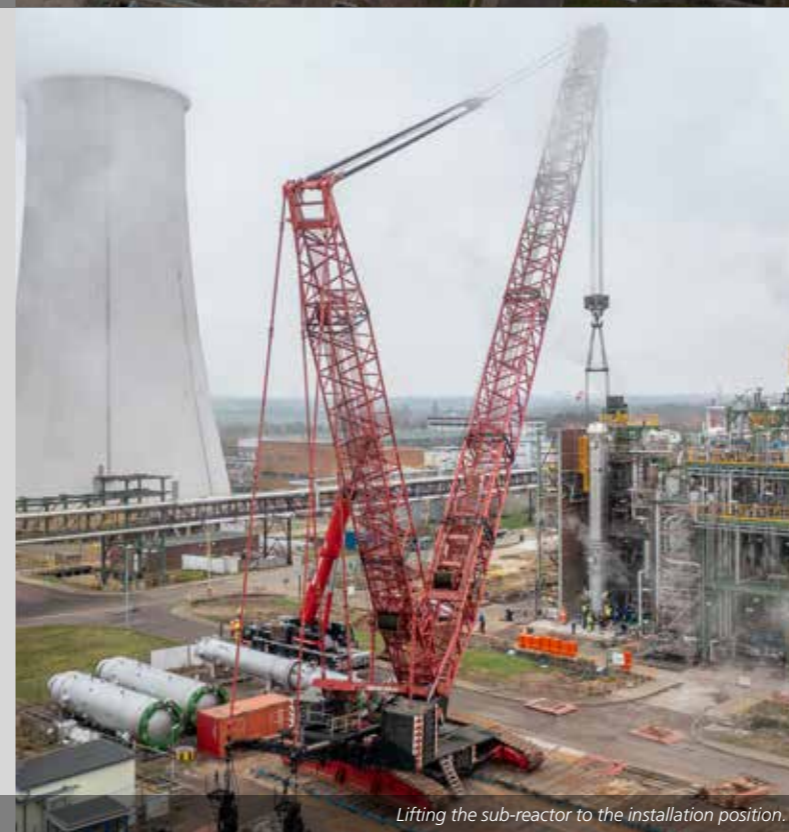
Pivoting the sub-reactor in the direction of the plant.
